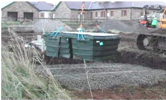
Figure 1 - Lifting Puraflo Module
