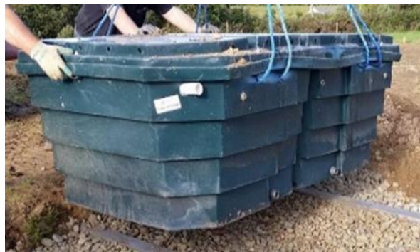
Figure 2 - Setting Puraflo Module in position
