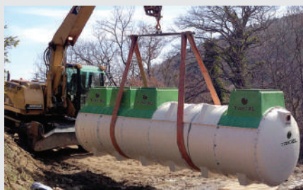
▶ Each wastewater treatment plant unit is constructed of lightweight SMC and is easy to manoeuvre which simplifies the installation process.
