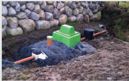
▶ Tricel Vitae 6 installed
