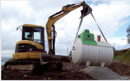
▶ Tricel Vitae 6 being installed
